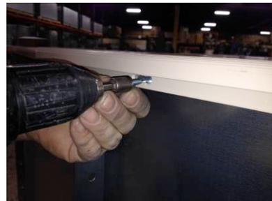
The PVC top seat also has a cap to cover the seams at each joint. This joint cap just snaps into place. Hook the back of the cap first then the front.
