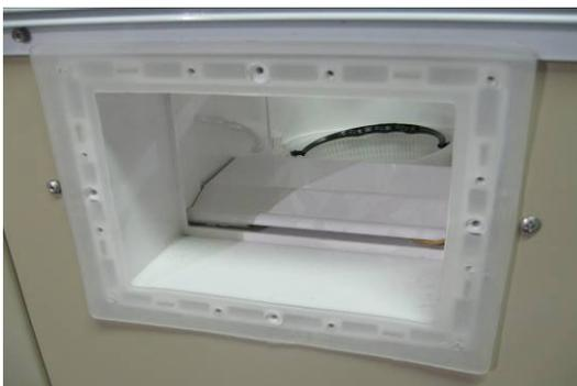
Before installing the liner, double check the pool walls and the pool bottom for any dirt or sharp objects that could damage the vinyl material. Last but not least, make sure the skimmer and return gaskets are in place.
