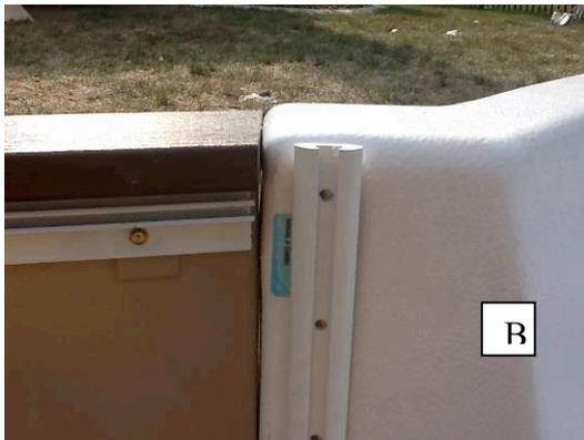
First locate the stair placement at the site. Insert the filler panel shown in photo “A”. Align the appropriate panels to either side of the stair and clamp them to the stair flange. When using the “synthetic wood” top seat or the “PVC coping”, the coping must be flush with the top of the stair as shown in photo B.
