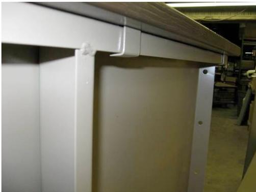
In your pool kit you will find sections of “dual track” white aluminum coping. To install the coping you will need your power drill and a 5/16 hex head socket bit. Each section of coping should be positioned tight against underside of the top seat and attached to the pool wall using the self drilling self tapping hex head screws. These screws should pass through both the coping and the top seat bracket.
