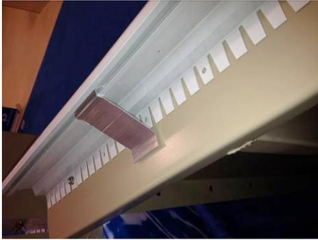
After the coping is mounted, place a support bracket, on the back side, in the middle of each panel and behind each coping joint. Lock the bracket into the back of the coping and fasten it to the top of the panel using one of the self drilling screws.
