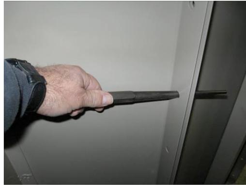
As you tighten the bolts make sure the panels are flush on the inside and the top seat joints are together. This will ensure a smooth liner installation and a flush top seat fit. Use a level to make sure that the pool walls are both plumb and level.
