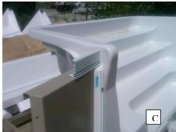
finished elevation is established, drill through the stair flange at each bolt hole location using a 1/2" drill bit and bolt together.
