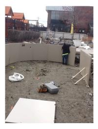
Secure the panels by using the 9/16" Galvanized nuts and bolts that were supplied with this package. Begin bolting the panels together using only the top two and the bottom bolt on each seam, until you have closed the circle. NOTE: Keep the panel connection on the outside of the layout stakes. We suggest that you hand tighten the panel bolts until the entire pool wall is erected.
