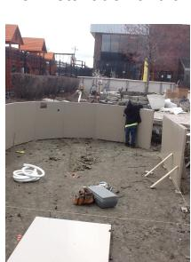
After the wall is assembled double check the position of the wall matching the wall seam to the perimeter layout stakes.
