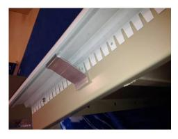
After the coping is mounted, place a support bracket, on the back side, in the middle of each panel and behind each coping joint. Lock the bracket into the back of the coping and fasten it to the top of the panel using one of the self drilling screws.
