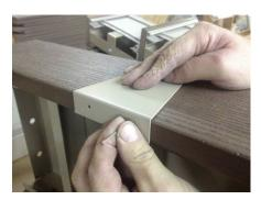
Locate the top cap joint covers and position them over each miter joint. Each cap hooks in the front first and secured to the top seat with color coated nails as shown.
