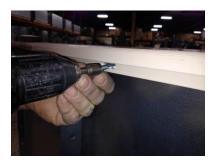
the self drilling 5/16 hex head self taping screws included in your pool hardware kit. These screws should be places no more that 12" apart on both the front and back side of the coping.
