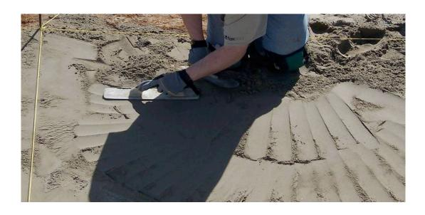
Spread the bottom material around the floor of the pool and compact it to just cover the string lines as you go. Use the edge of a flat board (about 36" long) to scrape the excess bottom material to expose the string lines. Run a trowel across the surface to smooth it out. A rounded bottom trowel works best. Remember to pull your pins and fill in their divots as you progress. "The last one out has to cover their tracks."
