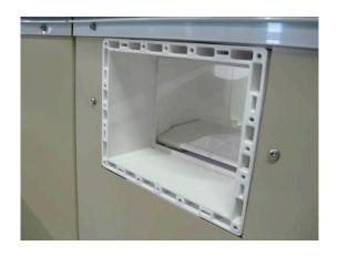
secure it using the two set screws supplied with the skimmer. If you have any questions, please refer to the manufactures installation instruction in the skimmer package.
