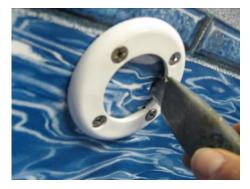
The return fitting face plate is installed in somewhat the manner as the skimmer. First find the round face plate and the pack of four faceplate screws supplied with the fitting.
