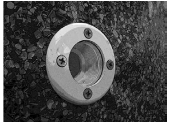
Return faceplate installed.
