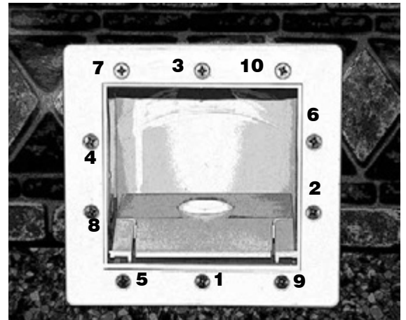
Skimmer faceplate installed w/screw tightening sequence.
