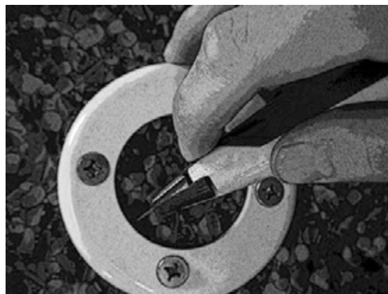
Trim liner from return opening.
