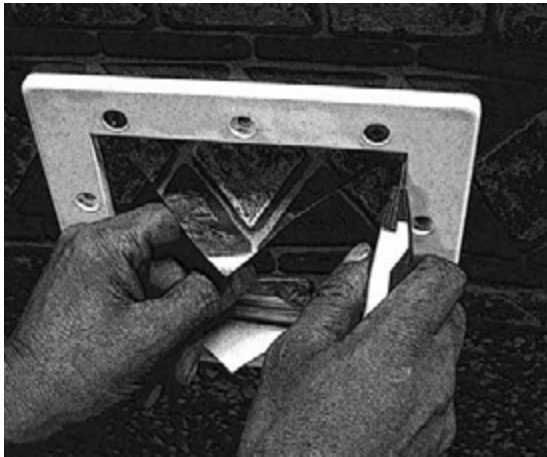
Trim liner from skimmer opening.
