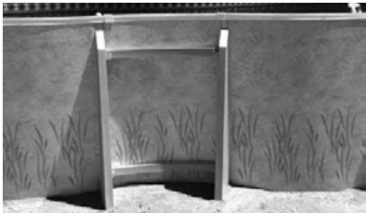
Aboveground with Structural Bracing
