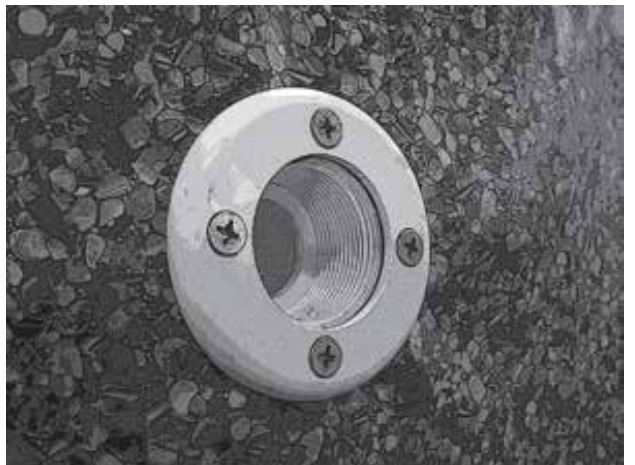
Return faceplate installed.
