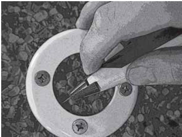
Trim liner from return opening.
