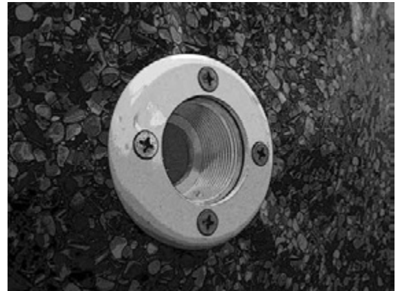
Return faceplate installed.
