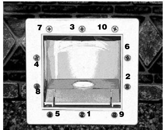
Skimmer faceplate installed w/screw tightening sequence.
